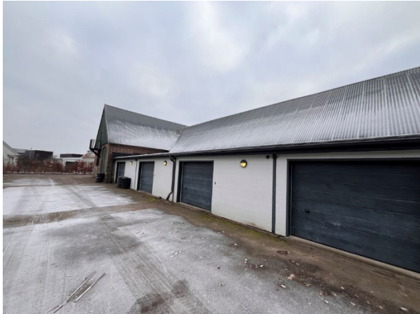
Foto, fasad (garage)
